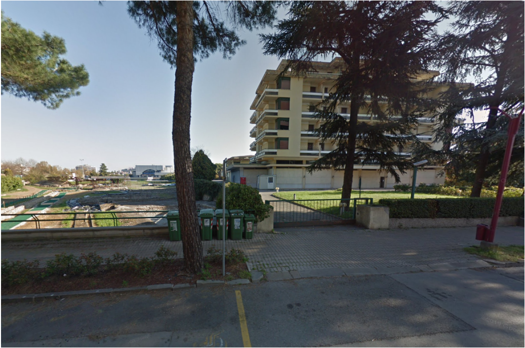
8 | View from Viale Stazione of the access road to Montecarlo Hotel bordering the archaeological area (photo by Authors, 2022).
